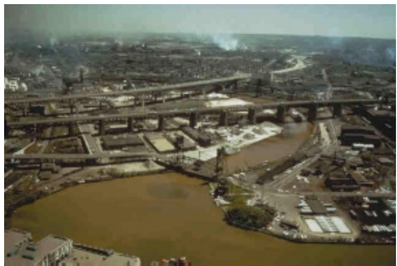
Contaminated sediments and other forms of industrial pollution continue to plague the Grand Calumet River.
