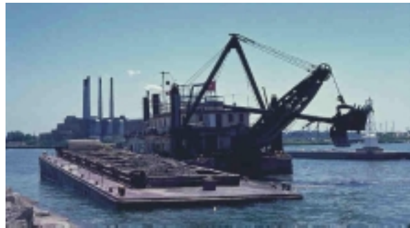
Dredging of the Grand Calumet is in process
